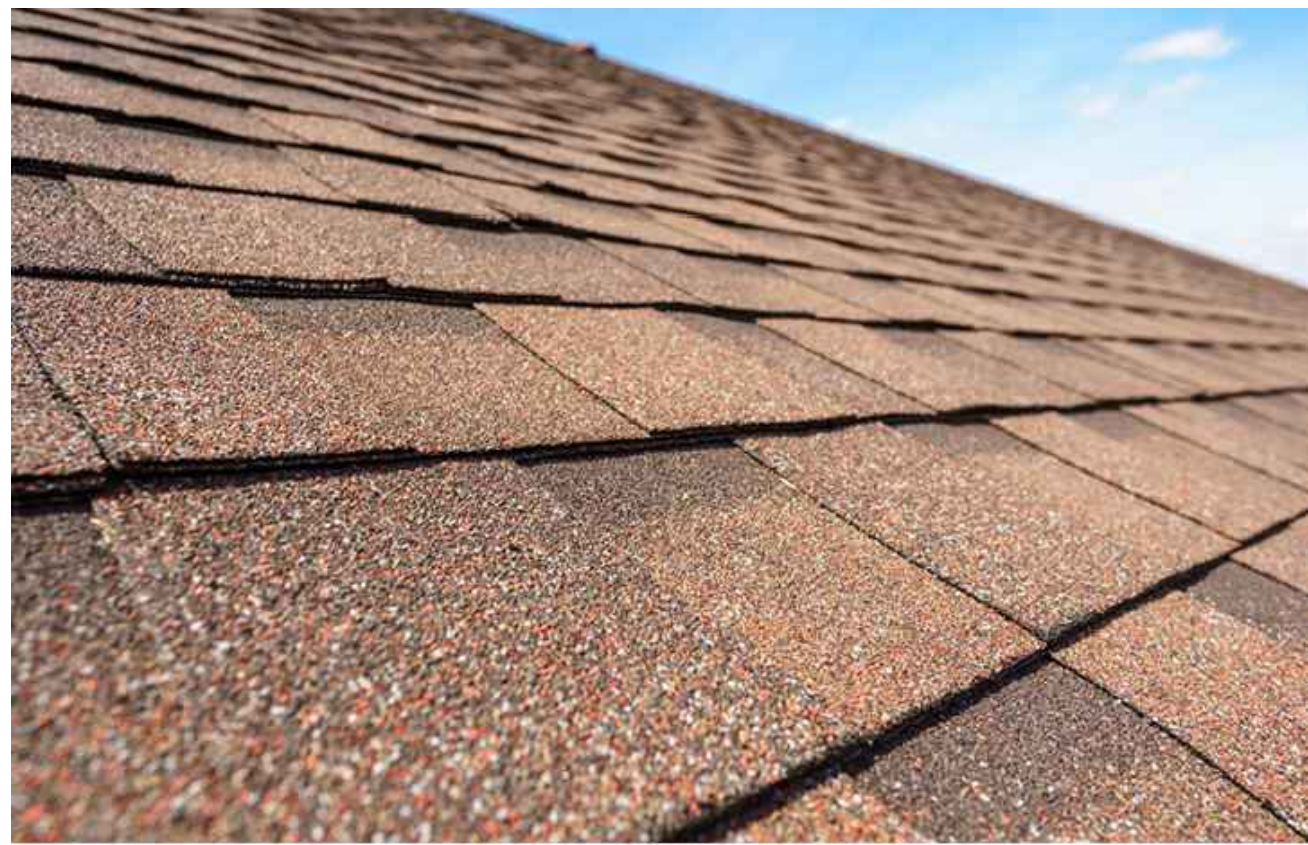
EXISTING ASPHALT SHINGLE ROOF TO REMAIN
