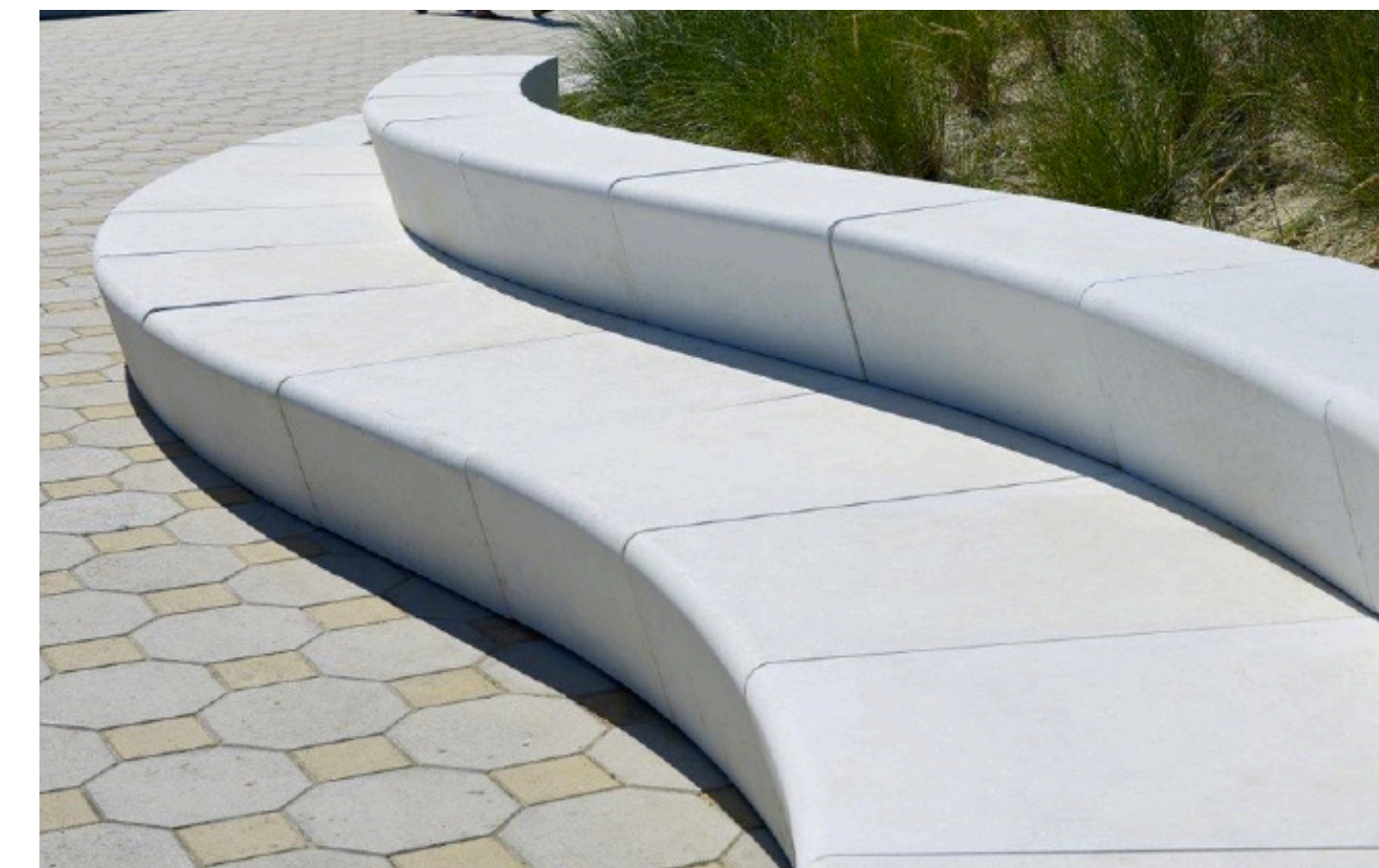
Concrete seat wall at splash pad area with 2-tier synthetic turf lounge terrace.
